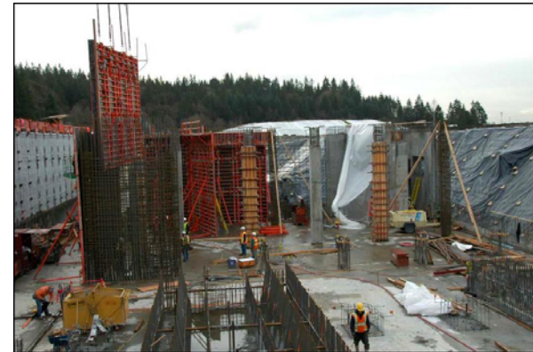
Brightwater Treatment Plant construction
