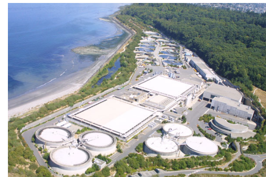
West Point Treatment Plant Seattle, Washington
