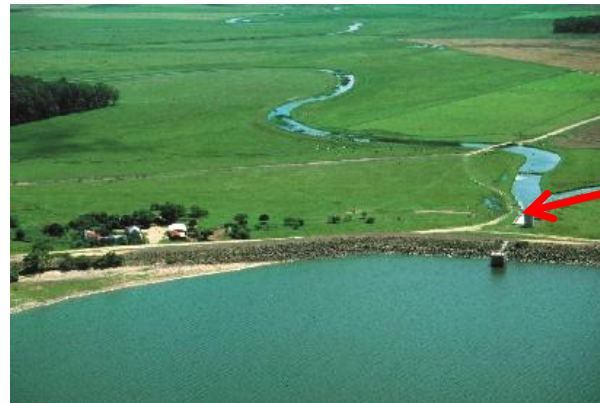
Existing irrigation dam
