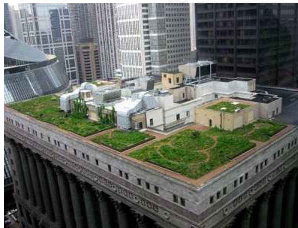
Figure 2: Chicago's City Hall Green Roof
