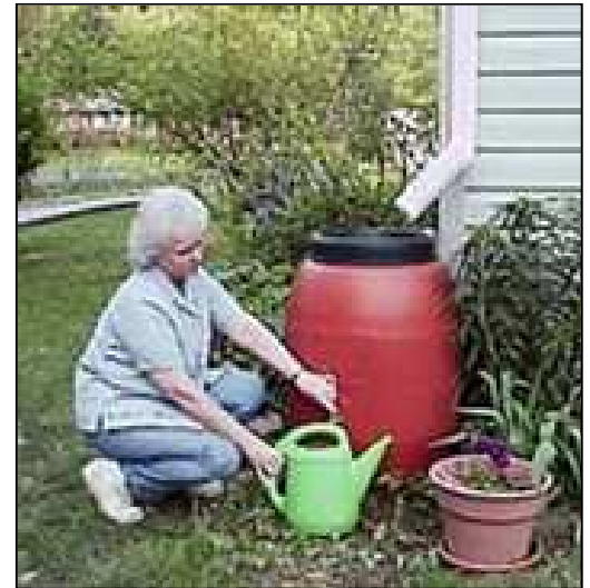
Figure 5: (Left) A gutter downspout connected to the storm drain system. (Right) A disconnected downspout using a rain barrel to collect stormwater for a rain garden
