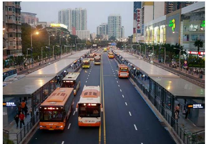
A key feature of the GZ-BRT is the segregated roadway lanes that allow the buses to run uninterrupted by private automobile traffic. These segregated lanes have integrated pedestrian walkways, metro stations, and bicycle lanes. Successful implementation was aided by several years of design, planning and analysis, with construction of all infrastructure, set-up of regulatory and operational systems, vehicle procurement and public outreach completed in 2009.
